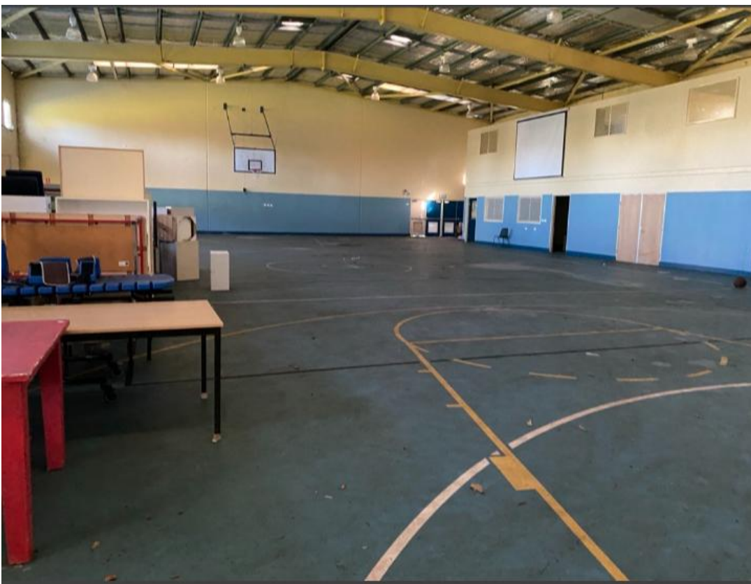
Figure 18 – Gymnasium to be refurbished internally
