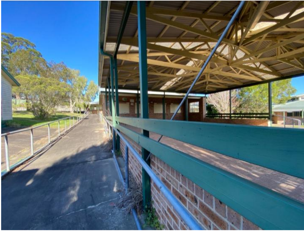
Figure 11 – Canteen to be demolished for car parking area
