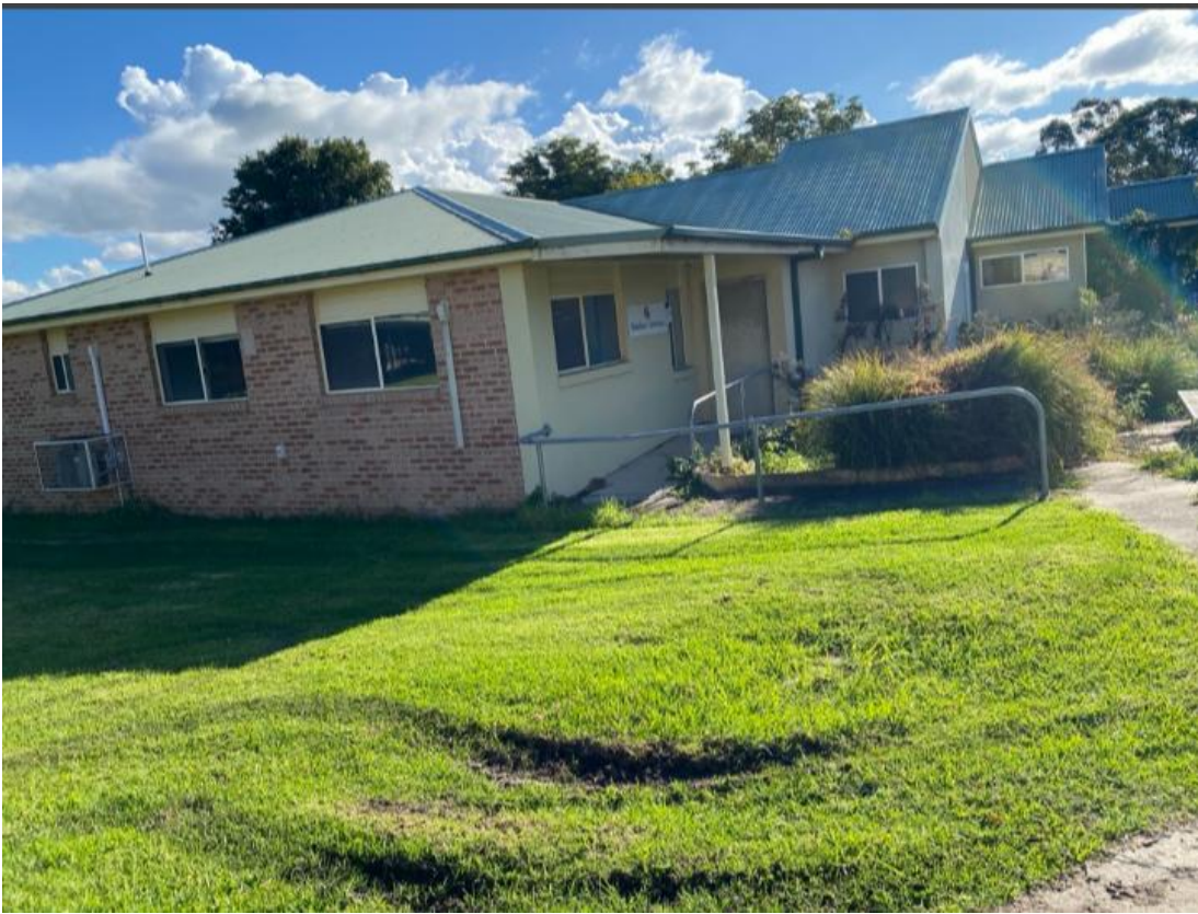
Figure 12 – Office building to be demolished
