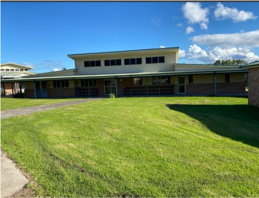
Figure 13 – Existing building “V” to be refurbished
