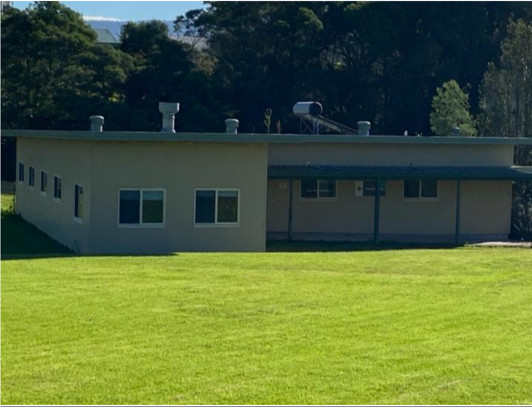
Figure 15 – Existing building “H” to be refurbished
