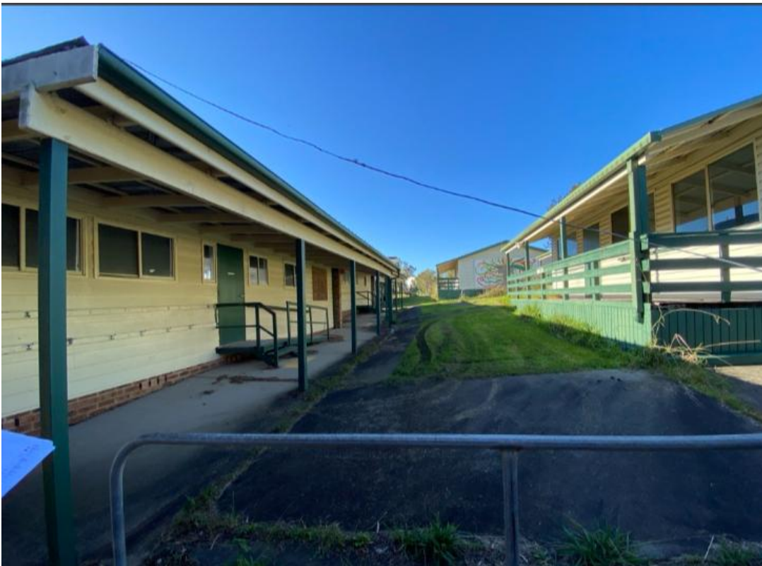
Figure 10 – Demountable buildings to be demolished for car parking area
