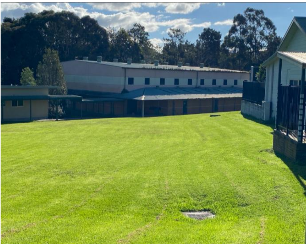
Figure 14 – Existing gymnasium building to be refurbished
