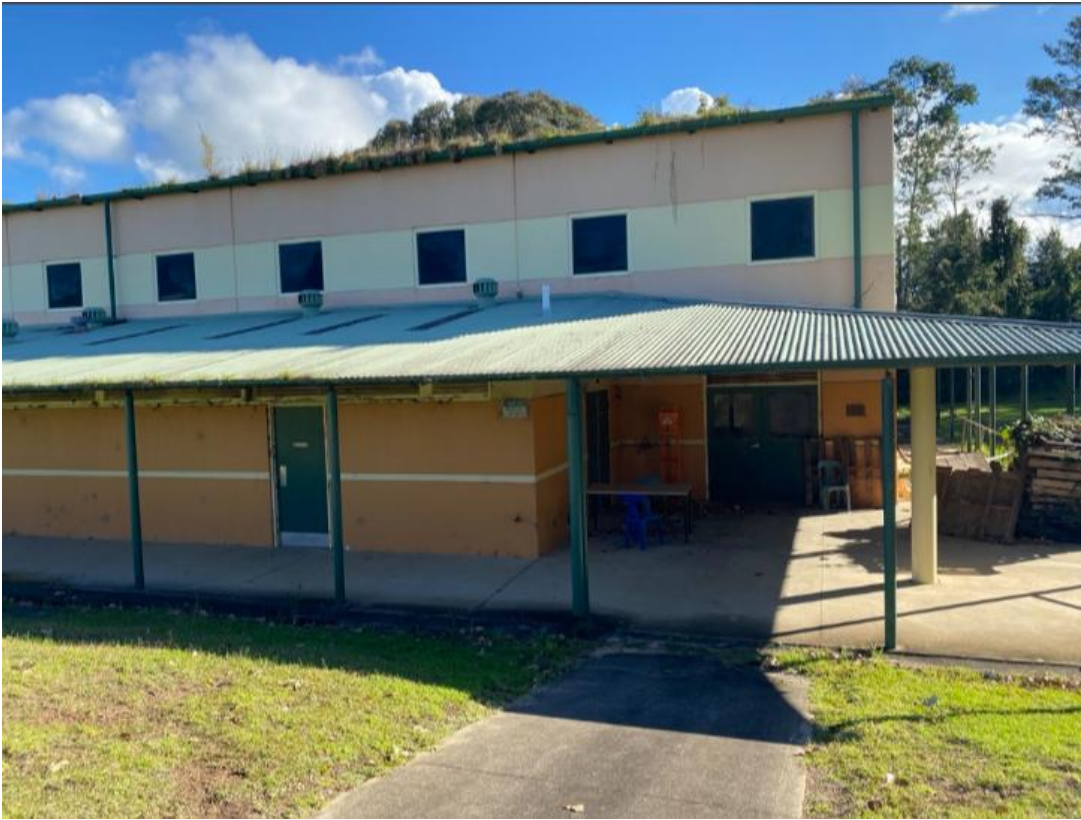
Figure 17 – Existing gymnasium building to be refurbished
