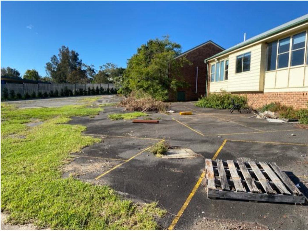
Figure 9 – Area and buildings to be demolished for new car parking area
